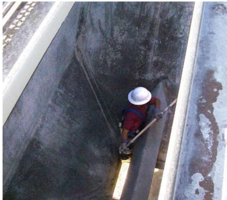
A Caterpillar skid steer does double duty, moving catchall bins under open hopper hatches and pulling along the air compressor (left). Inside the hopper, cleaning remains, in part, a hands-on job. A worker clears nooks and crannies with a hand scraper. Two photos: Carroll Group
